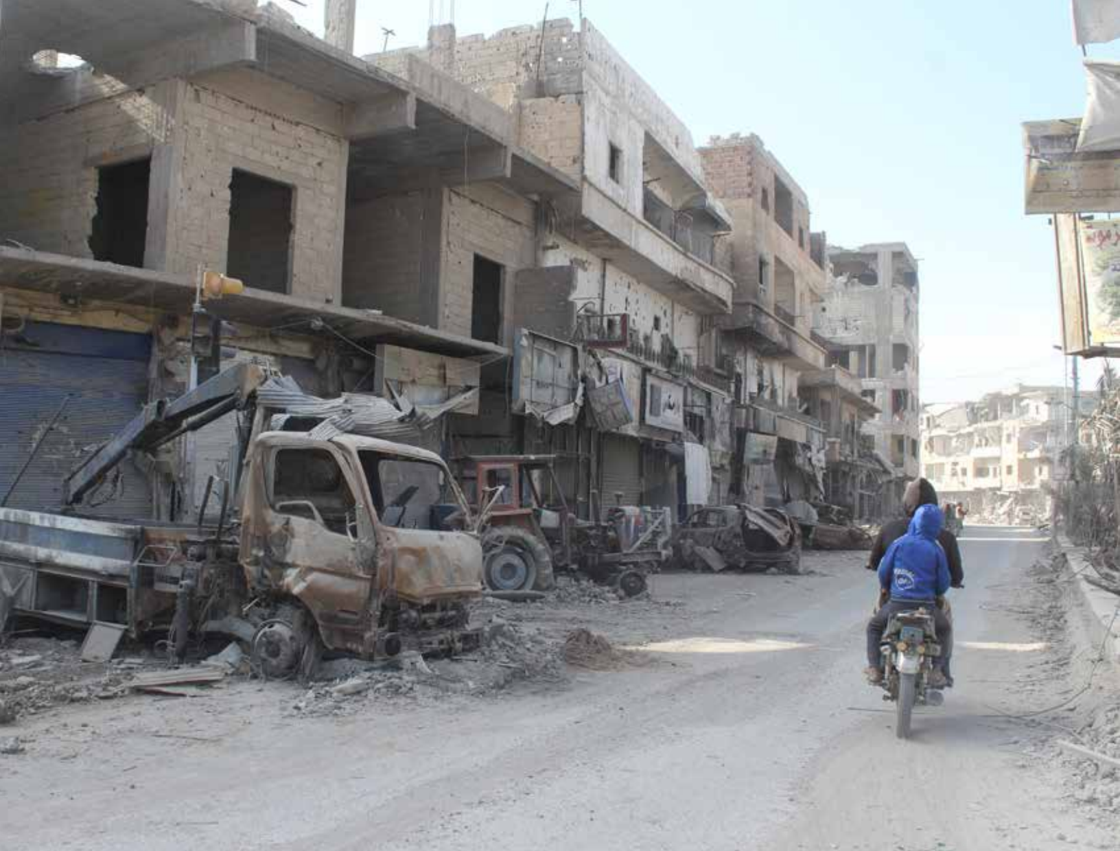
Damaged buildings in Raqqa, Syria. Numerous reports of civilian casualties emerged after a U.S.-led coalition and allied ground forces carried out a military offensive to clear ISIS from the city. December 18, 2017.
